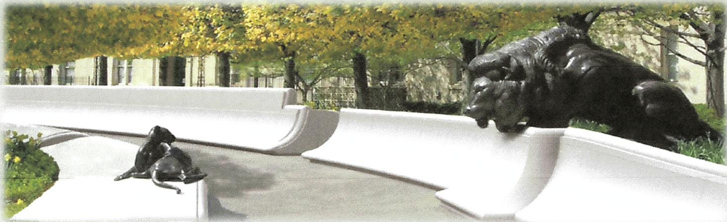
Architects designed a new 15" higher wall top-cap replacement that would add the needed space for names for another thirty-five years
